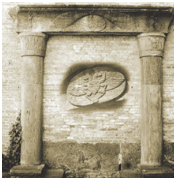
The rose-coloured sandstone portal is in the Ptolemaic style with two Egyptian columns having lotus capitals.
