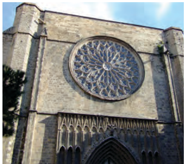
The two photos above are from Santa Maria del Pi, Barcelona (14 th Century). As with many early rose window designs, the structural strength of the wheel rim is clearly visible. This is unlike the more modern versions.
